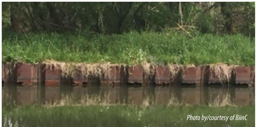
Medium size camp sheeting is generally constructed as so-called sheet-piling: interlocking profiles of tropical hard wood which are vertically installed into the soil using a vibrating hammer block. Tropical hard wood profiles used for camp
